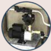
Pump pre-installed with rain/mains changeover
